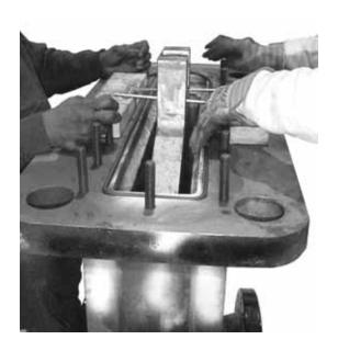
**6.1.17** Using proper equipment and lifting procedures, lift the entire top works assembly including the bonnet and slide the stem T-bar into the T-bar slot of the gate.
