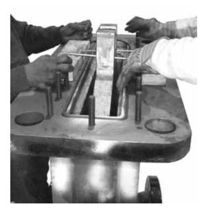
**5.8.25** Using proper equipment and lifting procedures, lift the entire top works assembly, including the bonnet, and place over the valve body.
